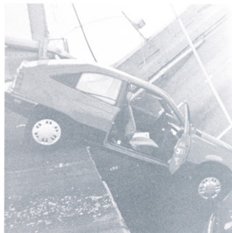
San Francisco Earthquake 1989
